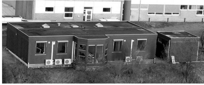
Figure 6. The PowerFlexHouse building.
